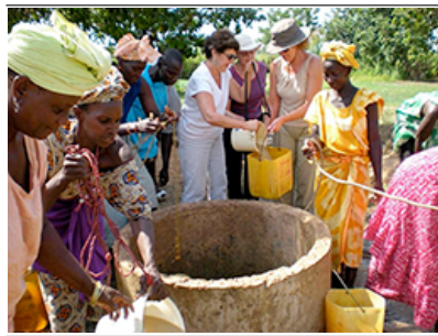
Finishing the well.
